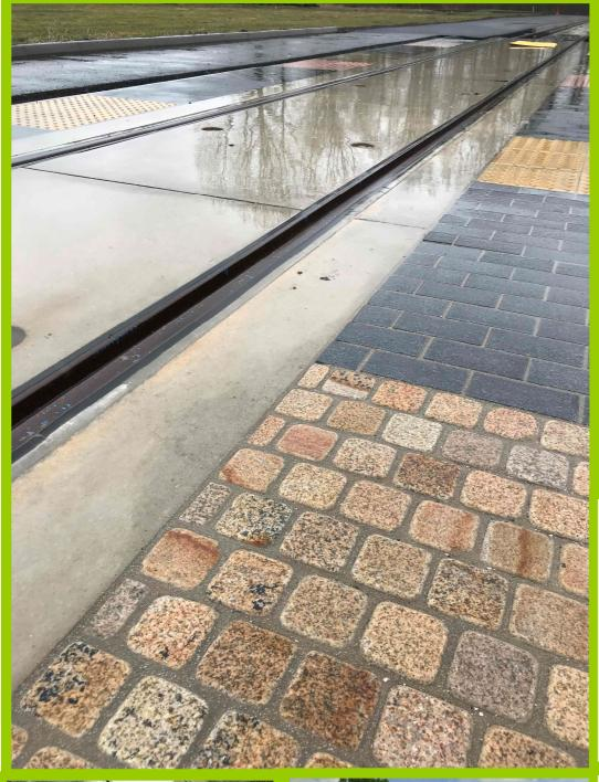
The high strength PCAT precast slabs reduces construction depth by over **50%**
