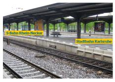
▲ Combined platforms in Karlsruhe: A 550mm platform is used for light rail services (left) and a 340mm platform for city trams (right).
