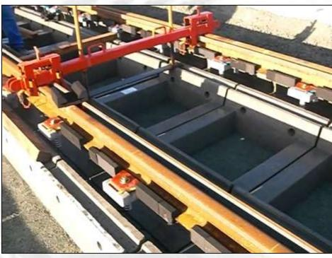
Installation of rails into precast element recess
